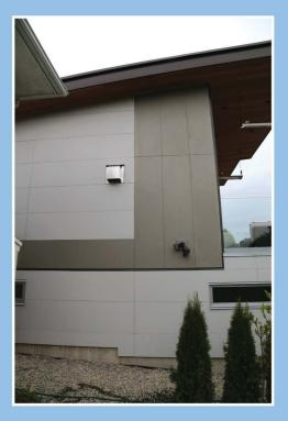
**Increased Safety:** MagO can easily be cut with a carbide saw blade, the dust has no carcinogens or toxins, much safer for the workers.
